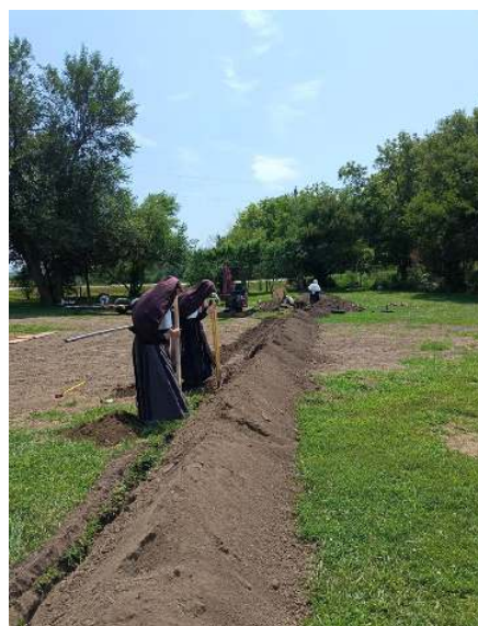
Digging for the electric line to our new chapel building
